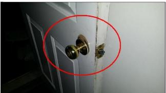
One or more door knobs and/or associated hardware are loose, damaged, stick or do not function properly. Recommend evaluation and repair by a qualified contractor.
