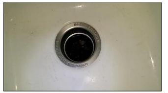
The rubber boot is damaged and should be replaced for safety and proper function. Recommend evaluation and repair by a qualified contractor.
