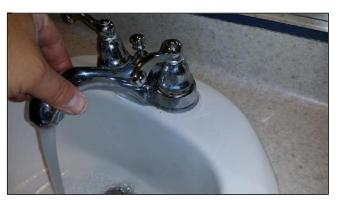
One or more faucets are loose and need to be properly tightened (upstairs hall). Recommend evaluation and repair by a qualified contactor.
