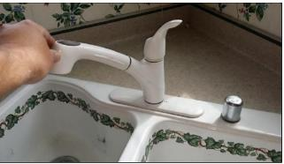
One or more faucets handles are loose and/or damaged. One or more faucet spouts are tight moving side to side. This could be from improper installation and/or some kind of damage. Recommend evaluation and repair by a qualified contactor.
