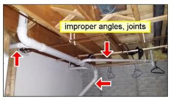
One or more pipes are in a non-standard configuration and are improper. Recommend evaluation and repair by a qualified plumbing contractor.
