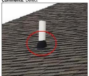
One or more pipe boot flashings are damaged. Recommend evaluation and repair by a qualified contractor.
