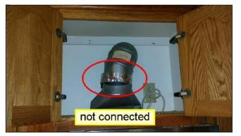
The exhaust duct work is damaged, not connected or not connected properly. Recommend evaluation and repair by a qualified contactor.
