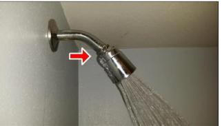
One or more shower heads are leaking. Recommend evaluation and repair by a qualified contractor.
