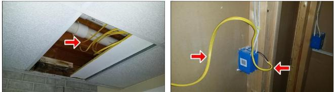
There are one or more improperly installed, supported or routed cables/conduits present. Recommend evaluation and repair by a qualified contractor.
