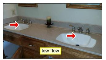
One or more faucets have significant reduced flow on hot and/or cold. The cause is not determined. Recommend evaluation and repair by a qualified contractor.
