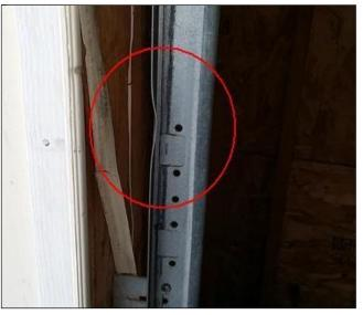
One or more door tracks are damaged. Recommend evaluation and repair by a qualified contractor.
