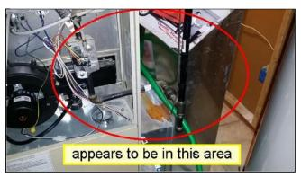
One or more gas supply pipes may be leaking. Recommend evaluation and repair by a qualified plumbing contractor.
