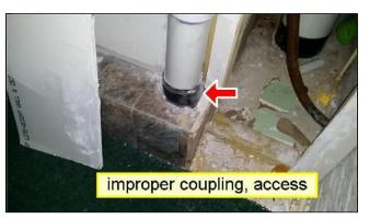
One or more pipes are in a non-standard configuration and are improper. Recommend evaluation and repair by a qualified plumbing contractor.
