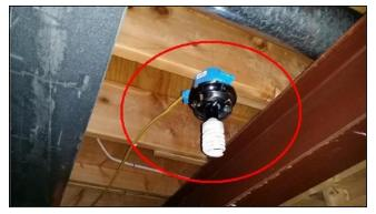
There are one or more lights that are damaged, improperly installed, not functioning or not functioning properly. Recommend evaluation and repair by a qualified contactor.
