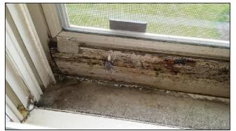
One or more storm windows are broken, cracked, damaged or have significant deterioration. Recommend evaluation and repair by a qualified contractor.
