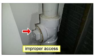
One or more clean out covers are not accessible. Remove the obstruction or move the cleanout. Recommend evaluation and repair by a qualified contactor.
