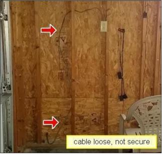
There are one or more damaged, improperly installed, supported or routed cables/conduits present. Recommend evaluation and repair by a qualified contractor.
