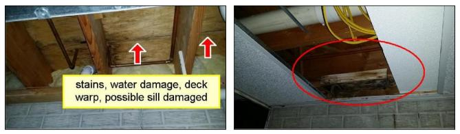
There is water damage present on the floor structure and/or sub-floor. Significant damage or weakening has occurred. Recommend evaluation and repair by a qualified contractor.
